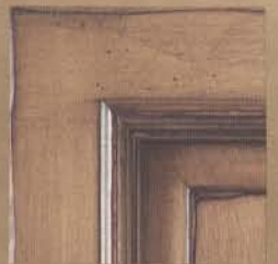
Heavy Distress & Rubthrough
